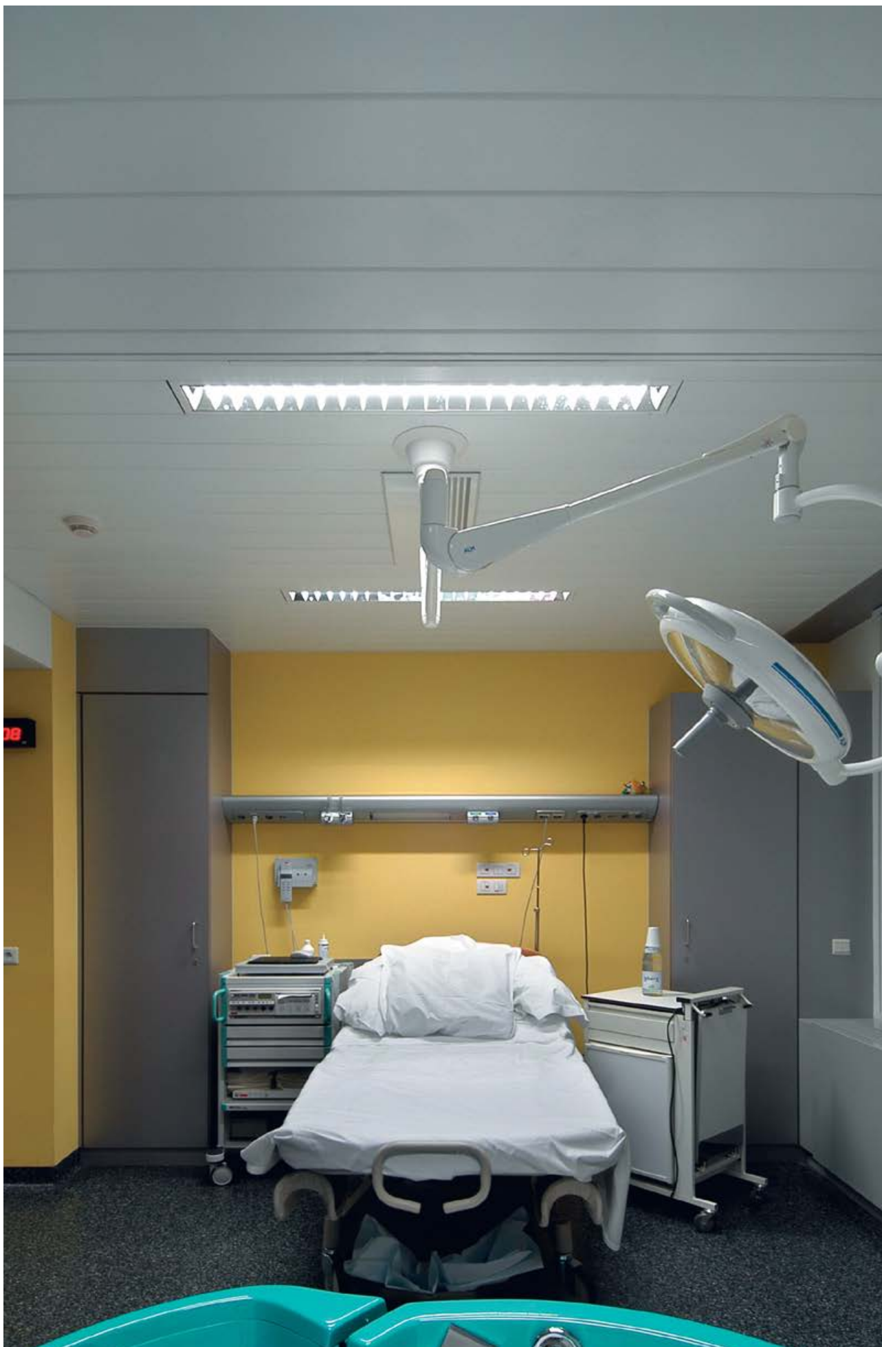
Project: Dodoens Hospital, Mechelen, Belgium - Product: Linear 225C - Architect: Luyten Lens
